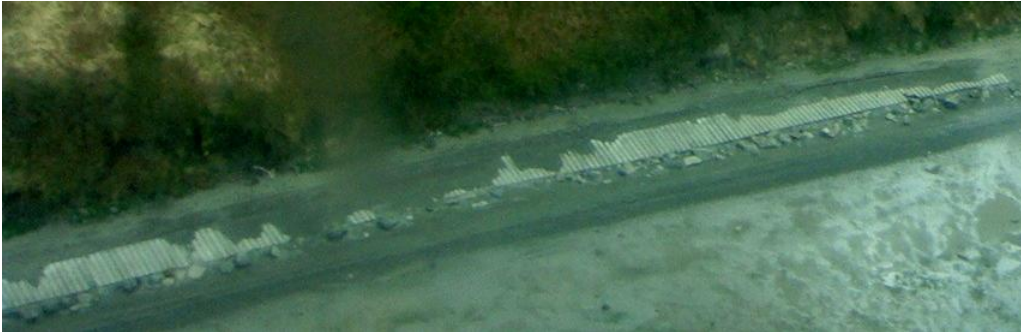
Figure 8: Existing road to Chignik Lagoon Landfill
