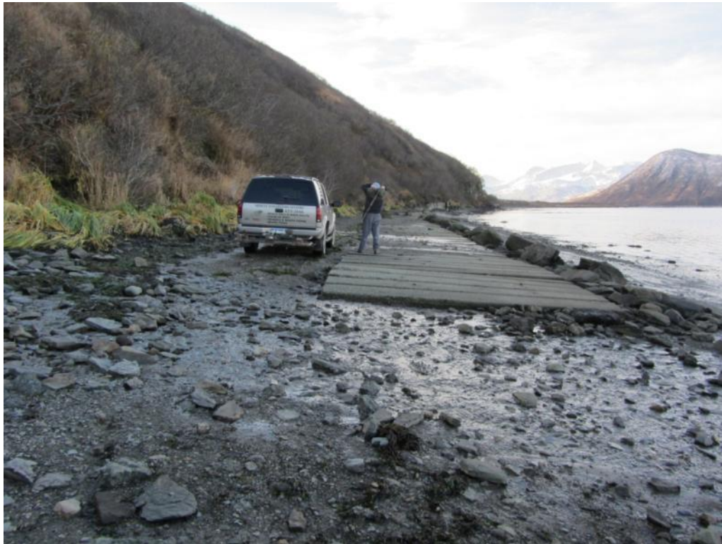
Photograph 6: Looking SSW along landfill access. Concrete road pads in foreground. Colluvium soil veneer overlaying bedrock is visible on hillside adjacent to shoreline.
