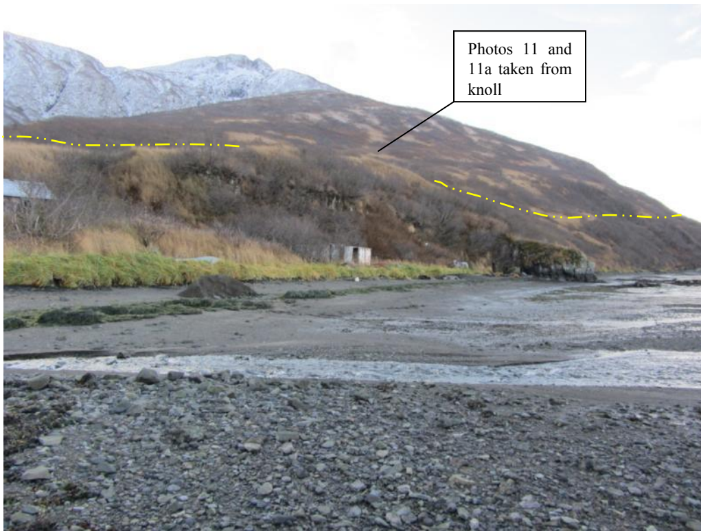
Photograph 5: Looking south at landfill access along shore from drainage outlet adjacent to Tract U. Proposed road alignment shown along hillside (yellow line).
