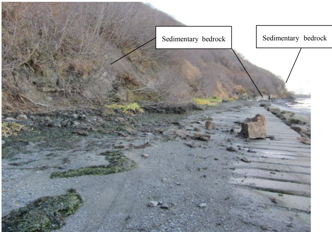
Photograph 7: Looking SSW along landfill access. Sedimentary bedrock exposed at toe of hillside. Bedrock exposed in cliffs in background.
