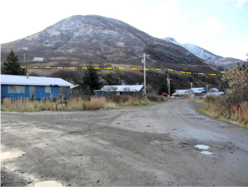
Photograph 1: Looking south east showing road alignment along structural bench above village
