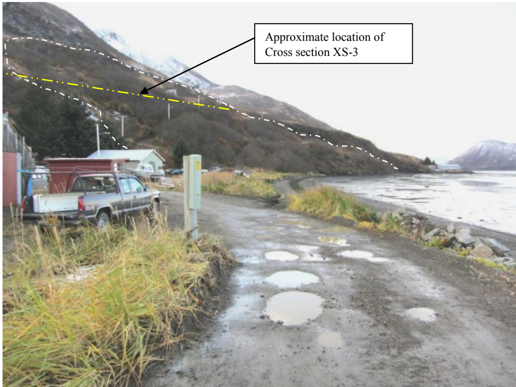
Photograph 2: Looking SE at road alignment (yellow line ) and ancient landslide area (white line).
