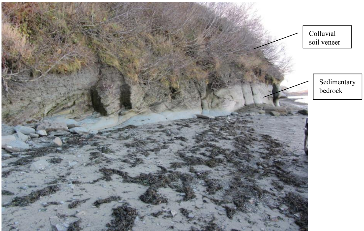
Photograph 8: Sedimentary rock outcrop with colluvial soil veneer along landfill access roadway (near station 664+00).
