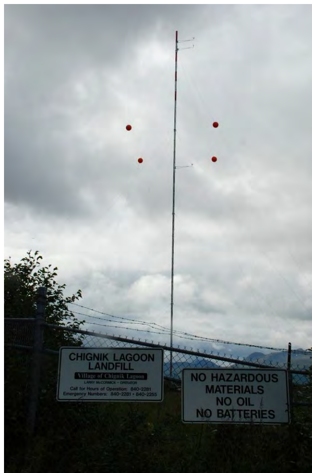
Figure 5. View of the tower fully erected.
